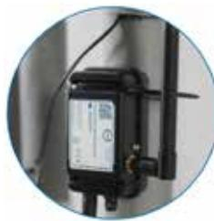
TMUs take temperature samples every 10 seconds (for hot, cold or blended supplies) and automatically begin recording additional data when outlet usage is detected.
