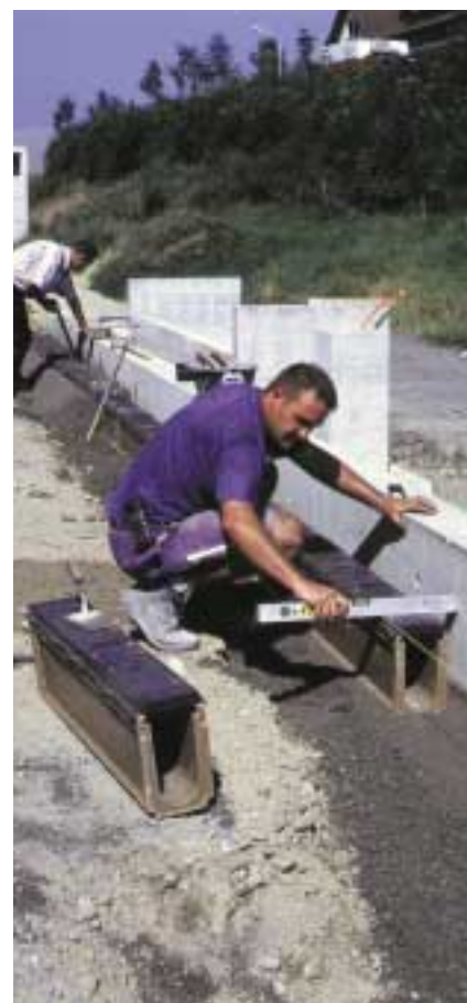
Channel installation
