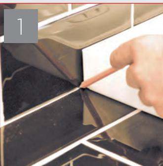
Lay the tray in position on the prepared floor and scribe a pencil line around the outside edge as in FIG 1 to mark the position of the tray, this will form the guide for the floor clips.
