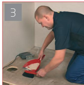
Prepare a rigid base of 10mm marine plywood, incorporating a suitable recess or cut out for the waste and fix to floor ensuring that the finished base is level and free of debris.
