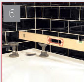
When all feet have been fitted level them up so that the base of the foot measures 95mm from the underside edge of the tray.
