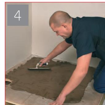
Cover the marine ply base with a 15mm depth of weak cement mix (sand / cement ratio 5:1).
