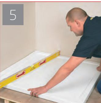
Place the shower tray with the fitted waste onto the cement bed and apply gentle pressure with the base of the hand to force the tray into position then finally level the tray and allow to set.
