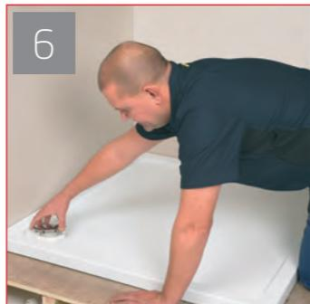
When shower tray is set remove the remainder of the protective film, connect the waste pipe and check for leakage.
