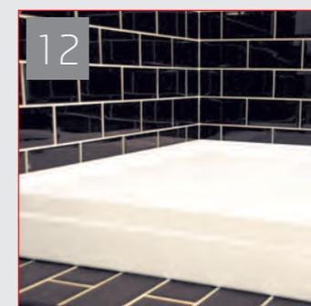
Fix the panels starting with the end panel or in the case of squares the panel with the rebated end by pushing firmly under the floor clips, then on to the adhesive pads and fix the front panel.
