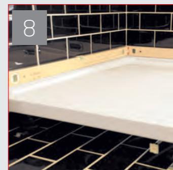
Turn the tray over and level both ways. When level fix the inaccessible legs with silicon sealer or no nails type of adhesive. Do not fix the central leg at this point. Screw the accessible legs to the floor, then adjust the central leg so that it forms a stabilising point.
