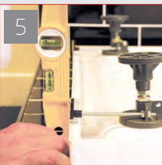
Fit the panel fixing rods, using a level. Ensure the face of the panel holder is lined up with outside edge of the tray as shown in FIG 5.
