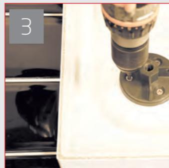
Screw the feet in position with the screws provided, if any are lost or missing use only the same size screws as those provided, 3/4 inch size 10 self tapping screw. Do not over tighten. Ensure you are using the correct foot that features the square web and holes for panel rods.
