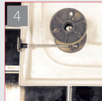
Ensure that the panel fixing holes are located at 90° to the edge of the tray as shown in FIG 4.
