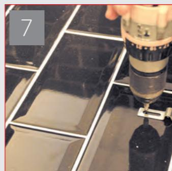
Screw down the floor fixing clips so that the edge of the clip is in line with pencil line made in FIG 1. Use all the clips provided and spread them equi-distant along both open sides of the tray.
