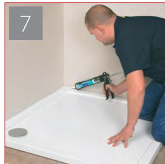
Seal joints between tray and wall with an anti fungi silicone sealant and allow to set, cover the tray with a soft dust sheet.
